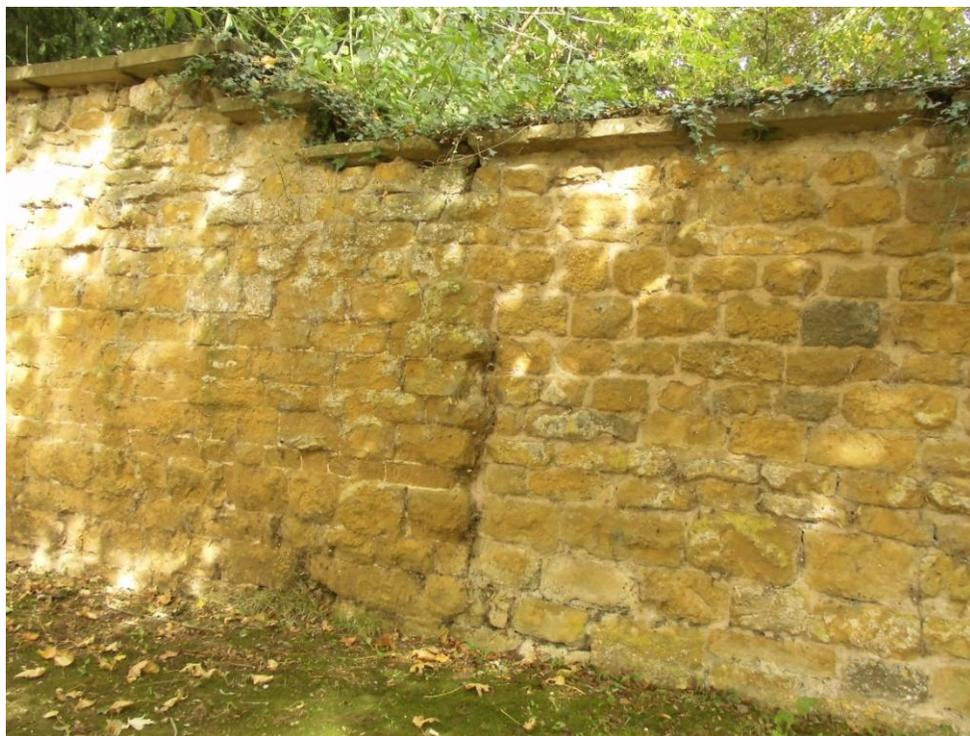
The large crack shown in the photograph above is just one of several signs of deterioration in the wall which separates the two village greens.
