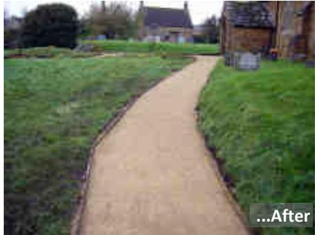
very similar to that used by the National Trust for their paths and has been approved by Cherwell. Gravel boards have been used to contain the gravel - over time they will blend in to give a natural edge to the path.
